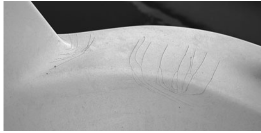
Small gelcoat cracks like this are mainly cosmetic. They can be filled, but may reappear again.
