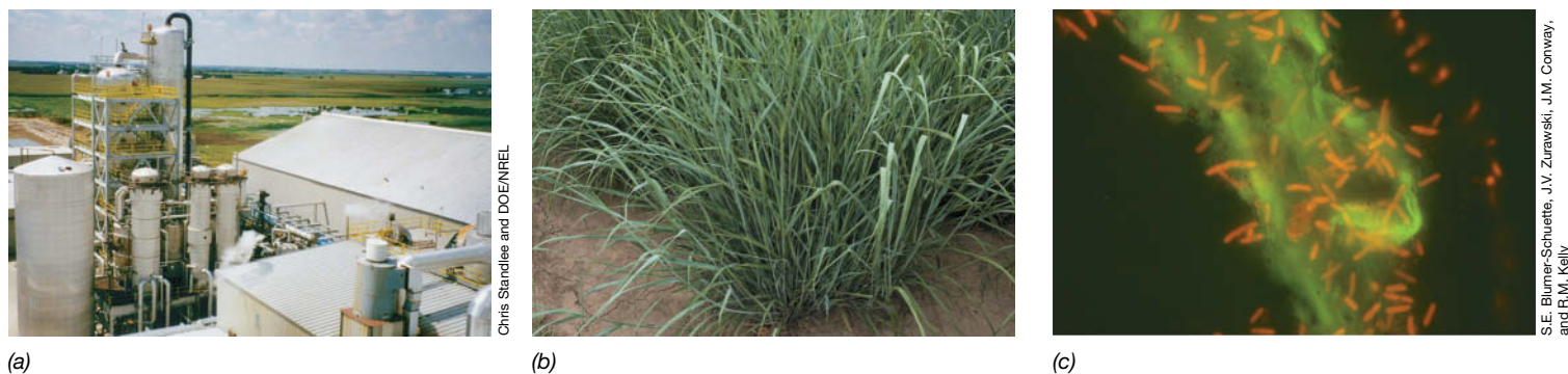
Figure 12.30 Biofuels. (a) A bioethanol plant in Nebraska (USA). In the plant, glucose from cornstarch is fermented by yeast to ethanol plus \text{CO}_2 . The large tank in the foreground is the ethanol storage tank, and the pipes in the background are for distilling the alcohol from the fermentation broth. (b) Switchgrass, a source of cellulose as a feedstock for ethanol production. (c) Fluorescence photomicrograph of acridine orange–stained cells of the thermophilic and cellulolytic bacterium Caldicellulosiruptor kronotskyensis growing on switchgrass (a single cell measures about 0.6 \mu\text{m} \times 3 \mu\text{m} ). The green color represents the switchgrass.
