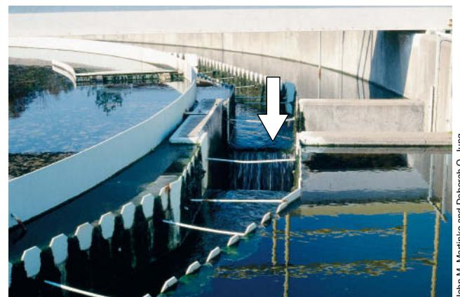
**Figure 22.14 Primary treatment of wastewater.** Wastewater is pumped into the reservoir (left) where solids settle. As the water level rises, the water spills through the grates to successively lower levels. Water at the lowest level, now virtually free of solids, enters the spillway (arrow) and is pumped to a secondary treatment facility.
