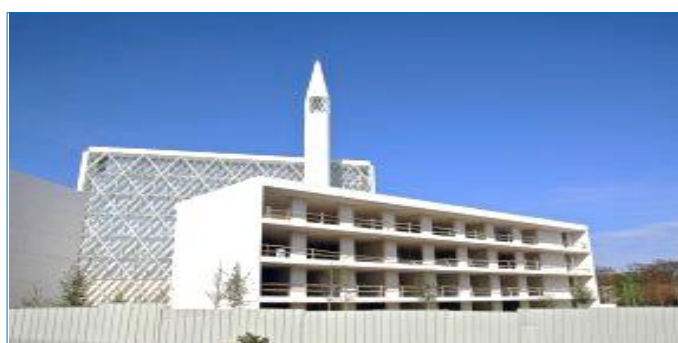
Figure 7: The mosque in Ljubljana, which is financed by Qatar. 20
